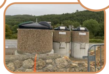
Containers semi-enterrés
